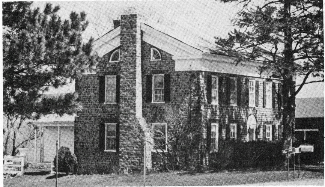
COLONIAL STYLE FARMHOUSE --One of the most elegant examples of early cobblestone architecture, 15545 Ridge Rd. W., where the Transit Rd. crosses, is the last cobblestone house in Murray, directly across from East Gaines. The large 10-room farmhouse is made up almost entirely of large and small fieldstones in random selection. At one period in the mid 1800's, this farmhouse was the home of Kurt Ruger and his 108-acre dairy farm. At present, it is the home of Mr. and Mrs. Lloyd Kuhns. Mrs. Kuhns is a charter member of the Cobblestone Society.
